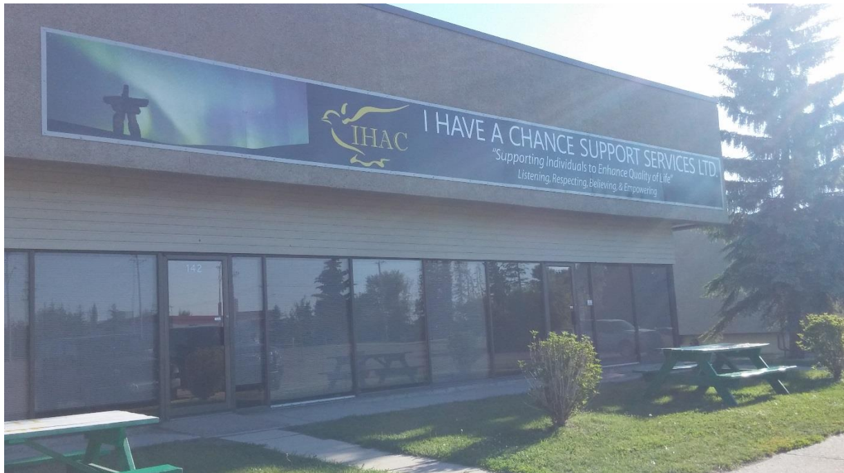
(IHAC Administration Office)
